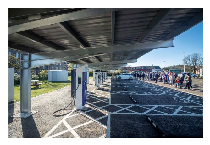
The chargers at this rapid charging hub consist of four rapid 50kW chargers and a 150kW ultra rapid charger for public use. DCC are intending to gradually introduce more 150kW chargers around the city in the future. There are also solar panels fixed to canopies which are positioned overhead and provide power to battery units on site which store this energy. These battery storage units contain 800kW of energy that can be consumed at the most suitable times, like when chargers are in regular use.
